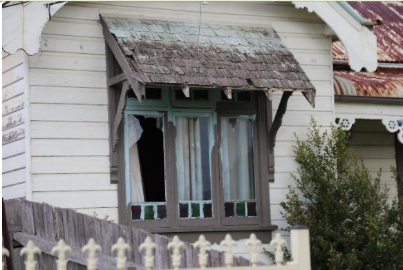
Detail of window to front elevation.
