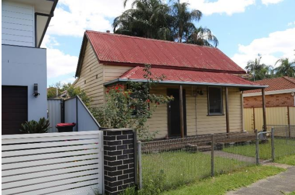
View northwest along Margaret Street to front façade.
