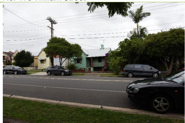
View to William Street Group.
