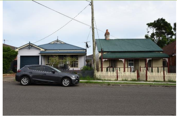
Overview of No. 28 and No. 30 Grimwood Street.
