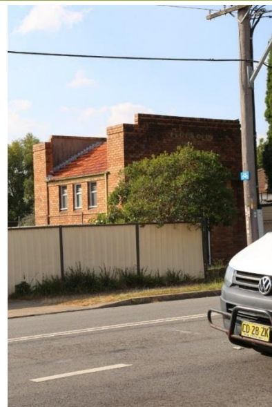
Front and western elevations of Substation.
