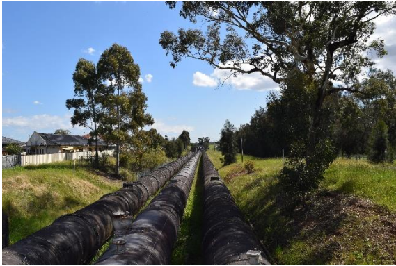
Figure 87. View northwest along the Pipelines from Barbers Road.
