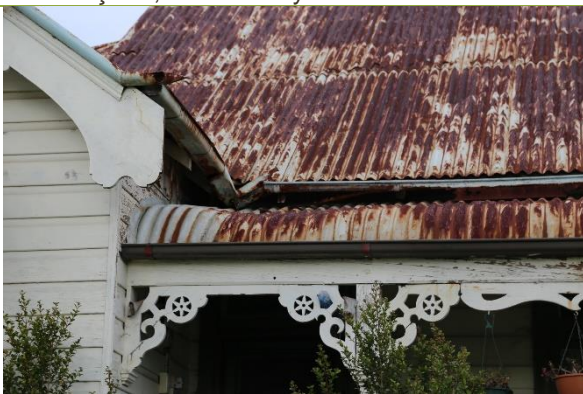
Detail of verandah and roof elements.
