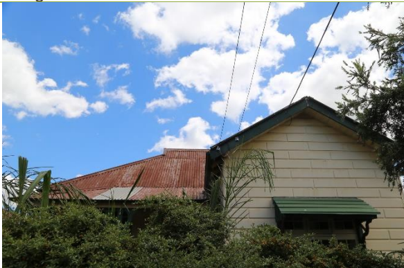
Detail of roof.
