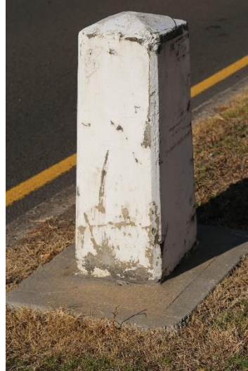
Merrylands Item 1 (Woodville Road, between Claremont Street and Patten Avenue).
