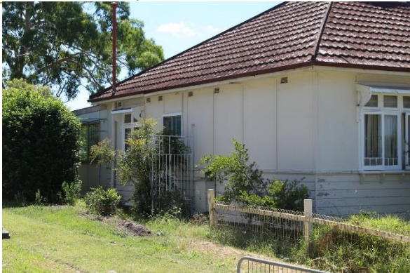
Southern elevation to cottage.
