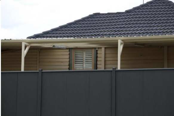
Detail to awning on western side of property.
