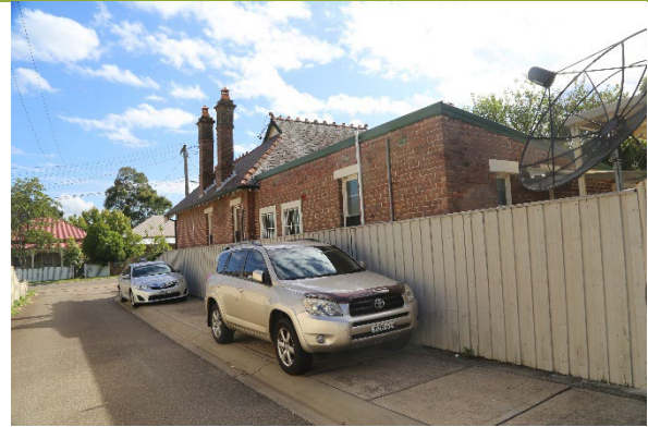
View north along laneway of west elevation.
