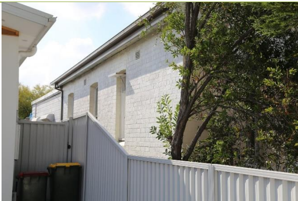
View to western elevation of cottage.
