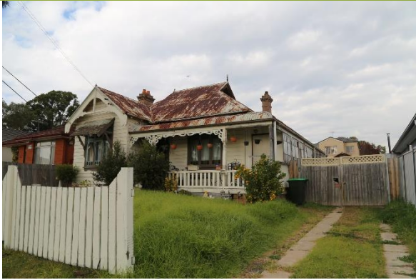
Front façade, fence and yard.
