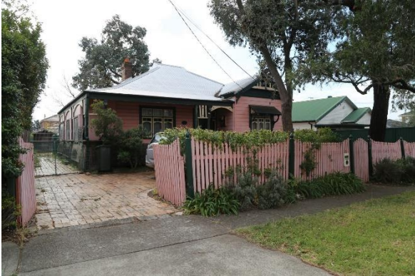
View from Earl Street showing the dwelling.
