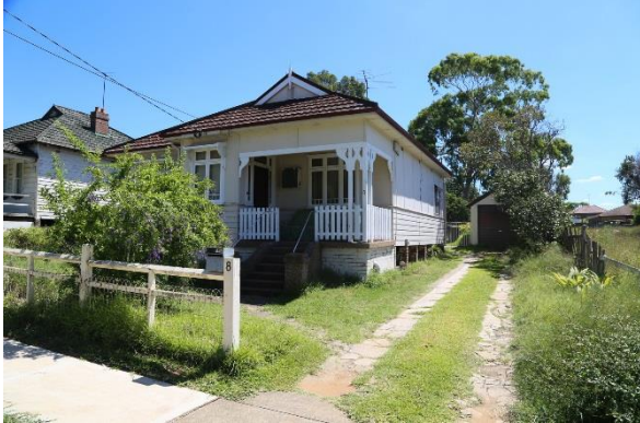
Façade and northern elevations of cottage.
