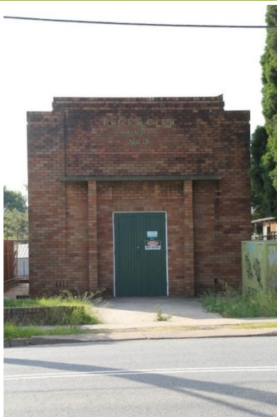
Electricity Substation from Guildford Road.
