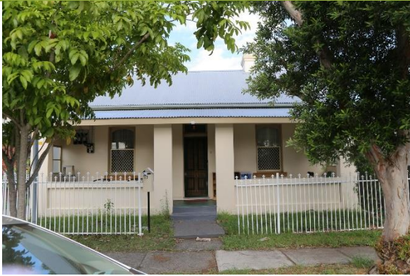
Front elevation and fence.
