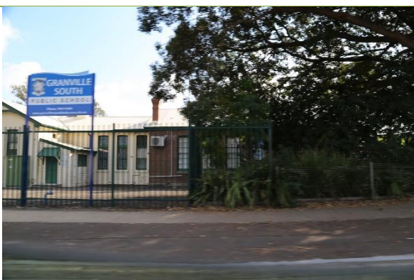
View to main building from Woodville Road, with 1902 brick extension.
