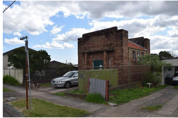
Figure 88. View northwest to the 'Electricity substation' (LEP ID I170).
