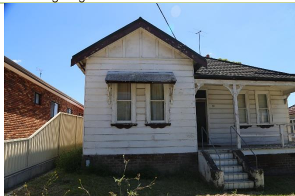
Overview of cottage.
