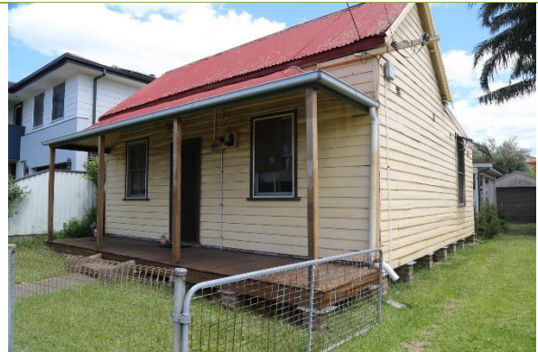
Detail of front façade and east elevation.
