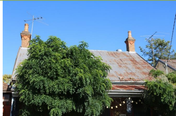
Detail of roof.
