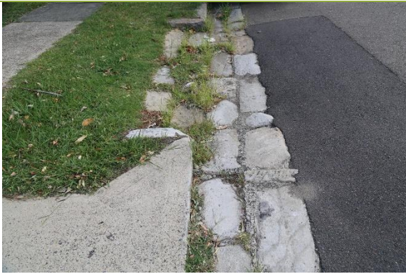
Detail of kerbing.
