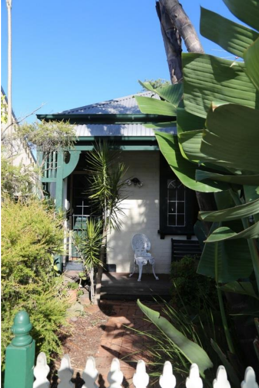
Detail of front façade.
