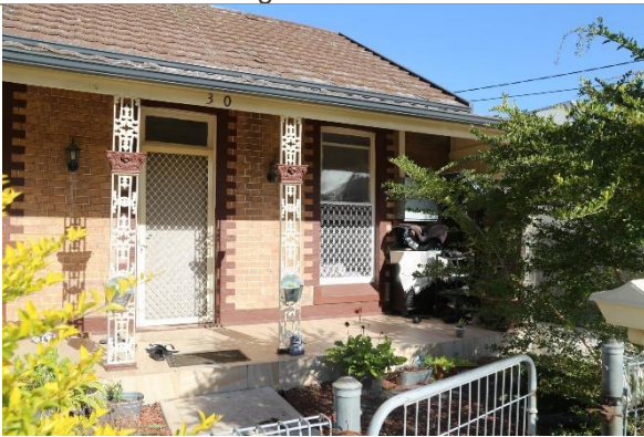
Detail of front façade.
