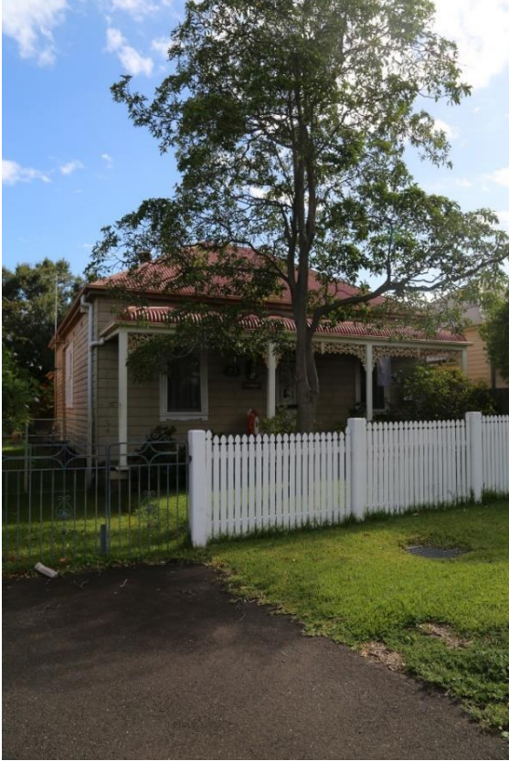
View to north elevation.
