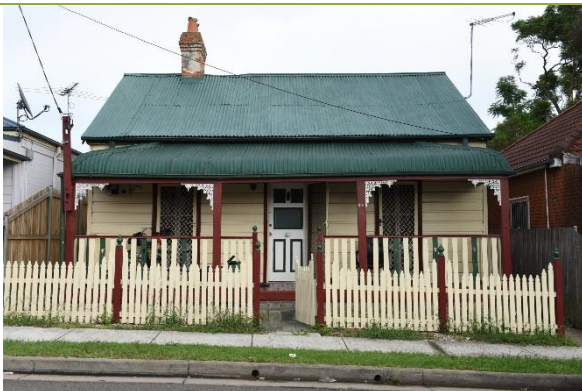
No. 28 Grimwood Street.
