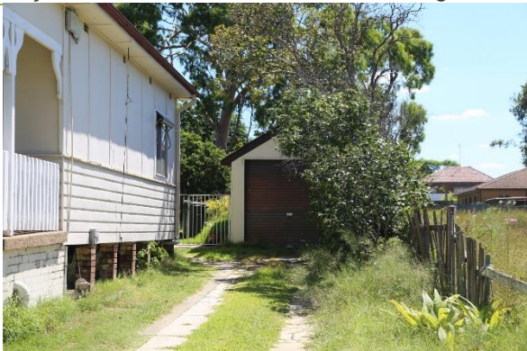
View of driveway and northern elevation.
