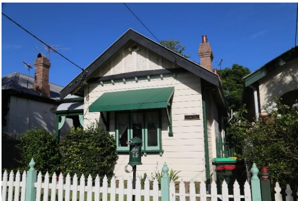
Detail of front elevation projecting gable.
