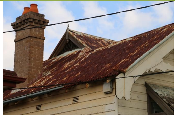
Detail of roof and chimney.
