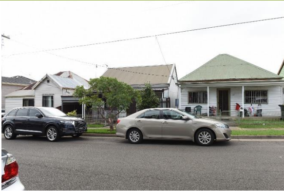
View to No. 23 and No.27 Grimwood Street.
