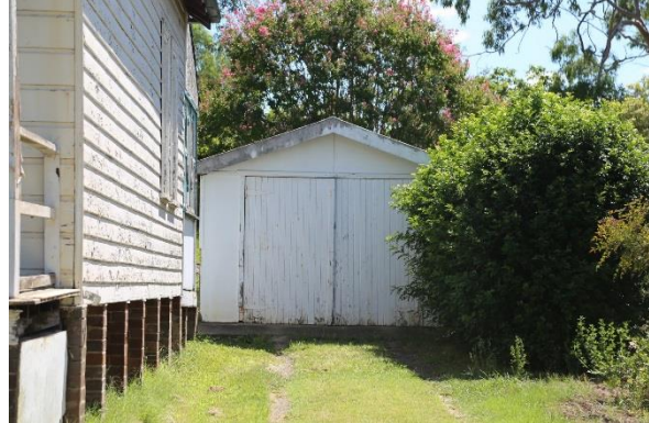
View to garage.
