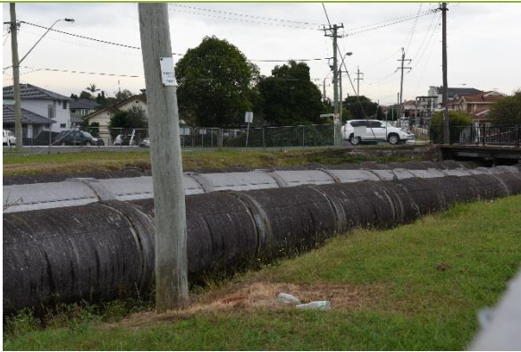
View of pipelines from Barbers Road, Guildford.
