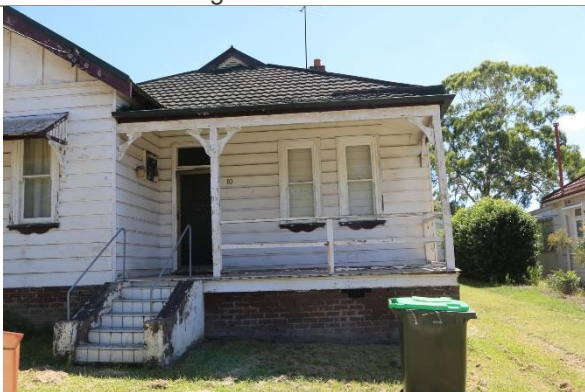
Detail to front verandah
