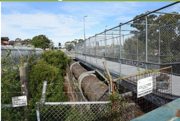
View of pipelines from Military Road, Guildford.
