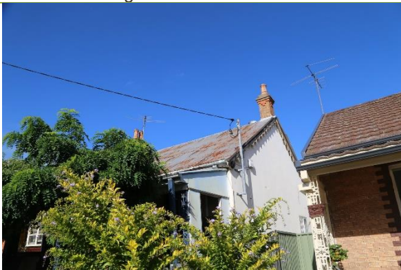
View of side (northern) elevation and roof.
