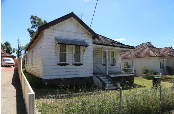
Overview of cottage.
