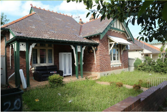
View looking east along Hewlett Street to front façade.
